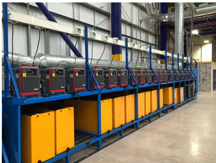
Triple Roller Stand & Charger Shelf Installation
