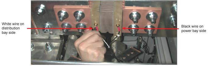
Figure 32 — Shunt Connections
