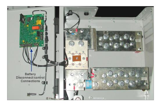
Figure 39 — Battery Disconnect Connections
