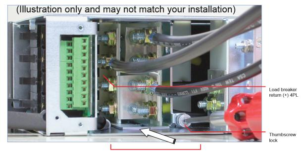
A Philips or slotted head screwdriver may be needed to secure the thumbscrew lock
