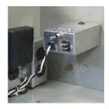
3. Connect SPI to power supply. For wiring instructions, refer to the XM Series 2 Technical Manual, which can be downloaded at www.alpha.com.
