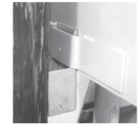
Fig. 6 Mounting the Lower Bracket for Wood Poles
