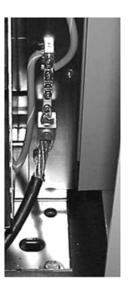
Fig. 3-4 System Grounding
