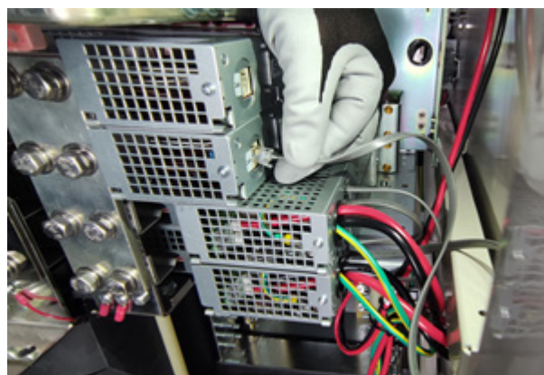
Figure 13: CAN cable installed to the lower hyperboost shelf
