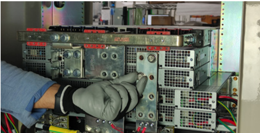
Figure 9: Spacer (not shown) with the –48 V link busbars installed to the right of the system
