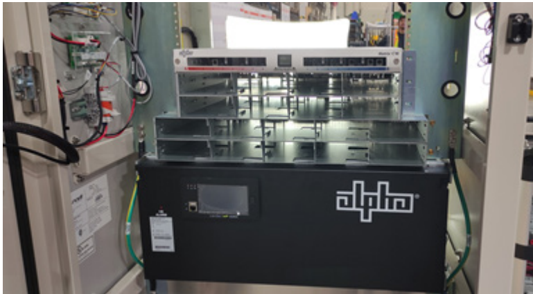
Figure 8: Cordex® CXPS-HSS hyperboost system on top of existing Cordex® CXPS-E6 edge power system
