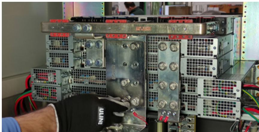
Figure 10: Common link busbar bracket installed on the middle of the system
