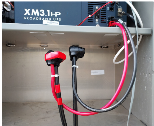
Fig. 4-16, Connecting 75A Anderson™ Connector
