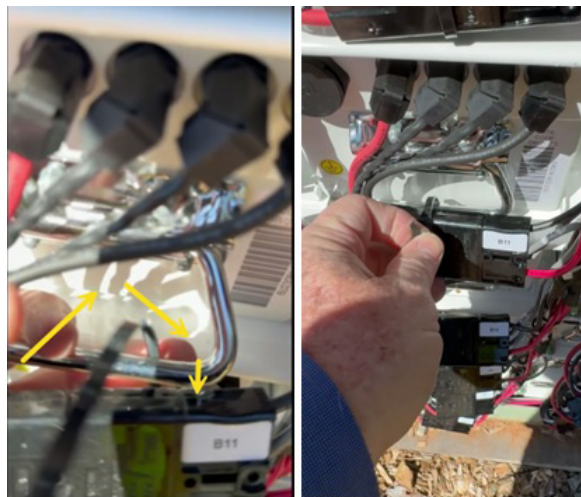
Fig. 5-26, Securing BPM Harness Connector
